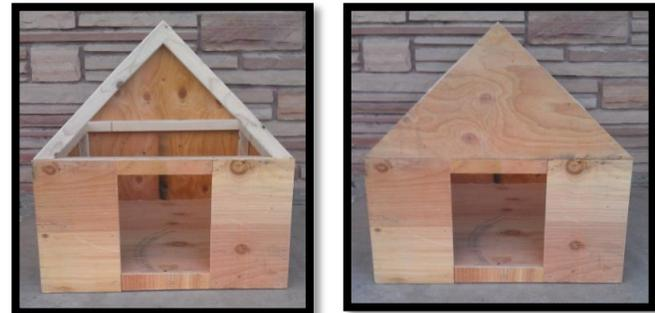
Picture 1 - Take the (2) Front Panels that measure 7-3/4" x 13-3/4" and screw them to the front of the dog house making sure that they are flush with the side wall.
