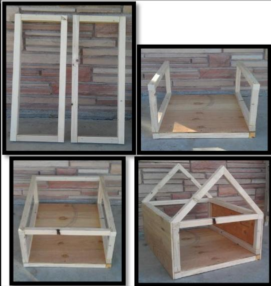
Picture 1 - Take (2) 9" (2x2's) and place them inside of (2) 30" (2x2's) to make a rectangle. Fasten the ends together using 2-1/2" screws. Do this step again.
