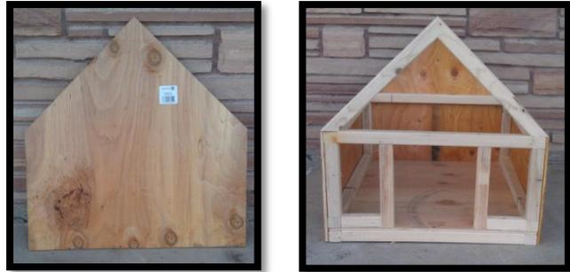
Picture 1 - Cut out back panel (6) and attach it to the back of the dog house. Make sure it's flush with the frame on all sides. Use multiple 1-1/2" screws.
