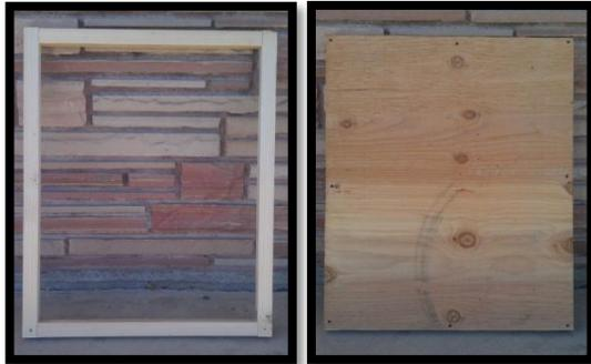
Take the 21-1/4" (2x2's) and place them inside of the 30" (2x2's) to make a rectangle that measures 24"x 30". Use 2-1/2" screws to fasten them together. Then place a 24"x30" piece of 3/8" CDX Plywood on top and fasten with 1" screws in multiple locations.
